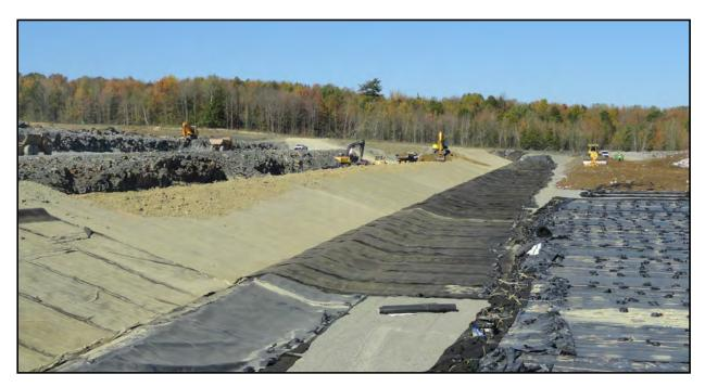
Photo 7: Cell 3-4 Berm Reconstruction
