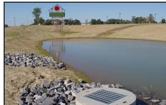
*Stormwater retention ponds, like this one under construction, provide effective Water Quality & Water Quantity Control in subdivisions and commercial developments.*
