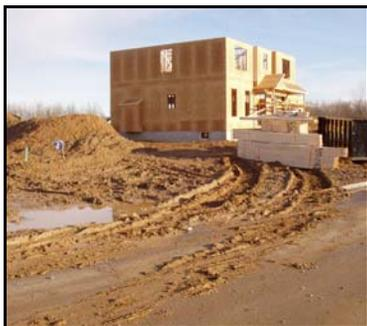
*Rain could easily wash this loose soil into the storm sewer and into a nearby stream, causing a water quality standards violation that could cost the site operator up to \$37,500 a day.*
